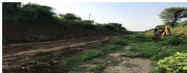
(FIG.3 ONE SIDE IS CLEANED/SHAPED AND OTHER IS UNDER MAINTANENCE)
