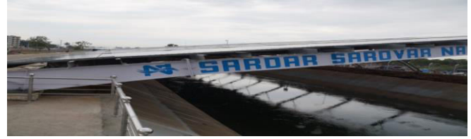
(FIG.6 SOLAR SYSTEM ON NARMDA CANAL, GUJRAT)
