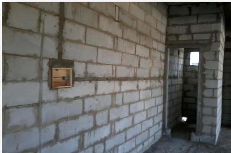
Figure 1.2 Construction of Autoclaved Aerated Concrete
