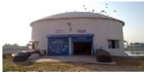
Fig.2 Pump House at Siddhi Sarovar
