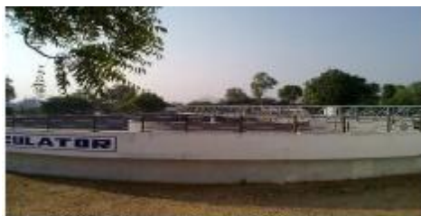
Fig.3 Water Treatment Plant at Siddhi Sarovar
